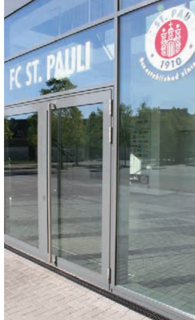
The ACO XtraDrain provides a permanently attractive effect and functionality. Above: The photo shows the facade channel on the stadium of St. Pauli Football Club in Hamburg
