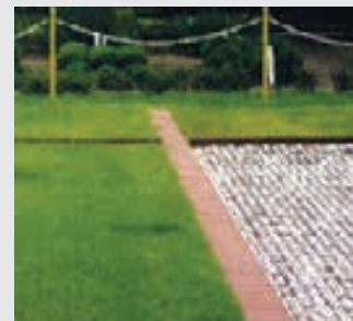
Parking space with Grass Grid (left) and chippings (right)
