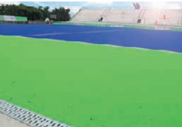
The hockey facility of the Olympic Games 2016 in Rio is equipped with ACO drainage channels
